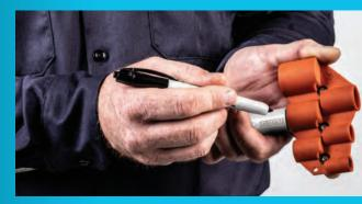
Step 3 Mark the pipe using the depth gauge tool
