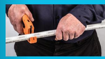
Step 1 Cut the desired length of pipe. • Square cut, perpendicular to length of tubing
