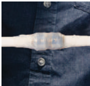
Finish by continuing to wrap 1" past the fitting.
