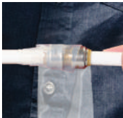
Wrap entire fitting, making sure to overlap each wrap a minimum of 1/4".
