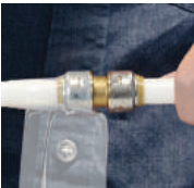
Start wrapping 1" before the fitting.
